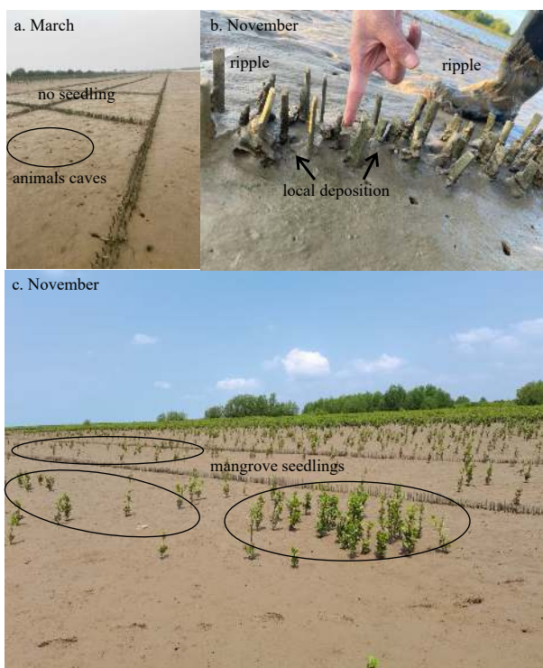
Fig. 11. View of bamboo fences contributed to animal habitat (a), sediment deposition (b), and mangrove expansion (c) so far.
